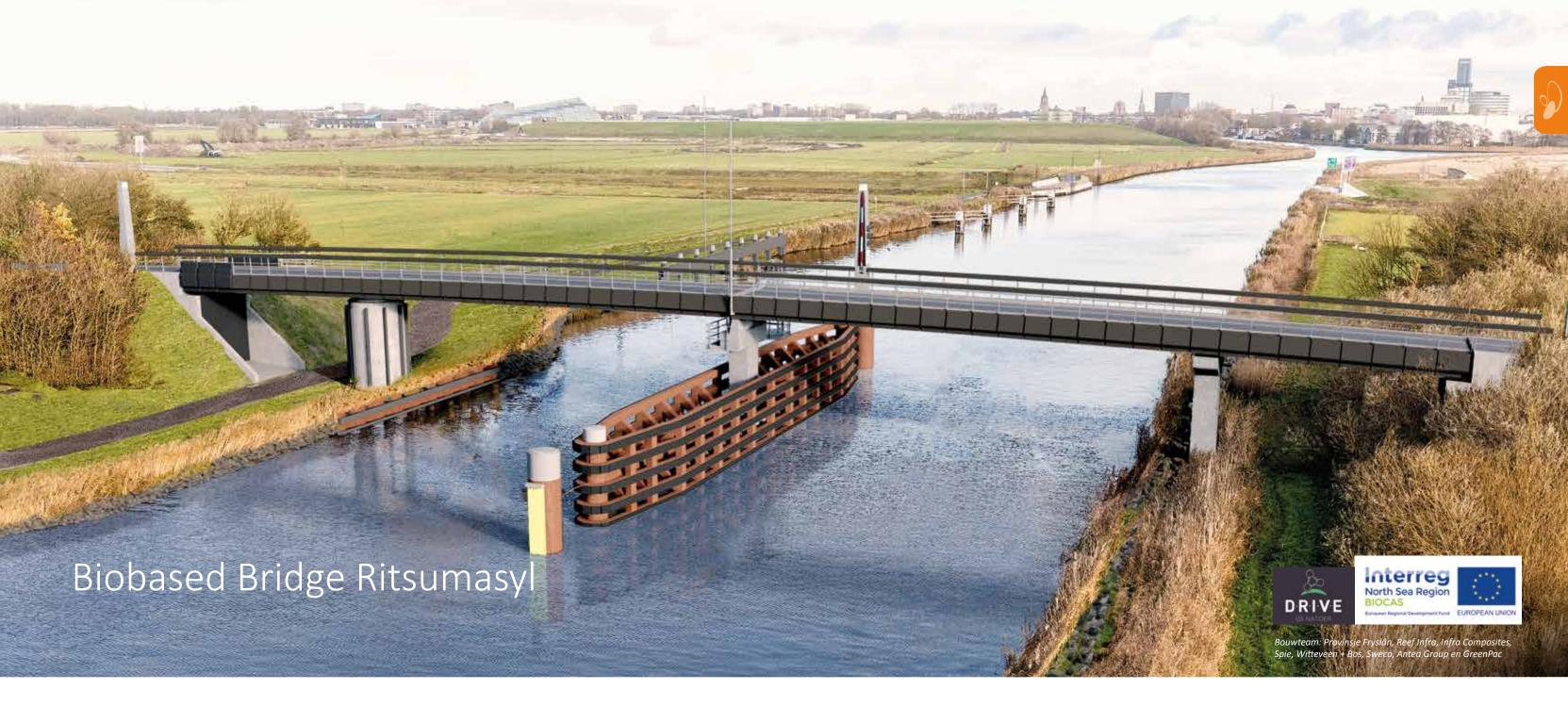
A movable bicycle bridge made of composites derived from organic materials is being built over the Van Harinxmakanaal close to Ritsumasyl in the northern Dutch province of Friesland. This biobased composite bridge — the first in the public road system in the Netherlands — is 66 meters in length, with a moving section stretching out over 34 meters and a fixed section of 32 meters.
